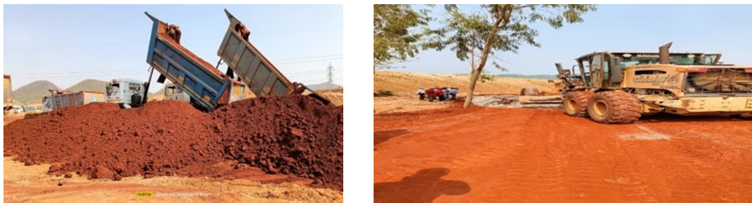
Figure 4. Dumping and in-situ mixing of red mud and fly ash of red mud at the pilot Site.
