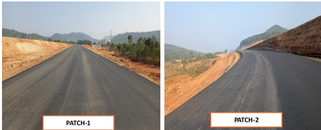
Figure 9. Experimental chainage 289 & 290, post bituminous concrete layer (BC).
