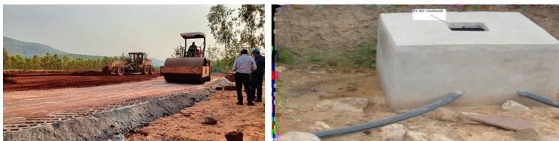
Figure 5. Left: Compaction of the subgrade section, Right: leachate collection chamber.
