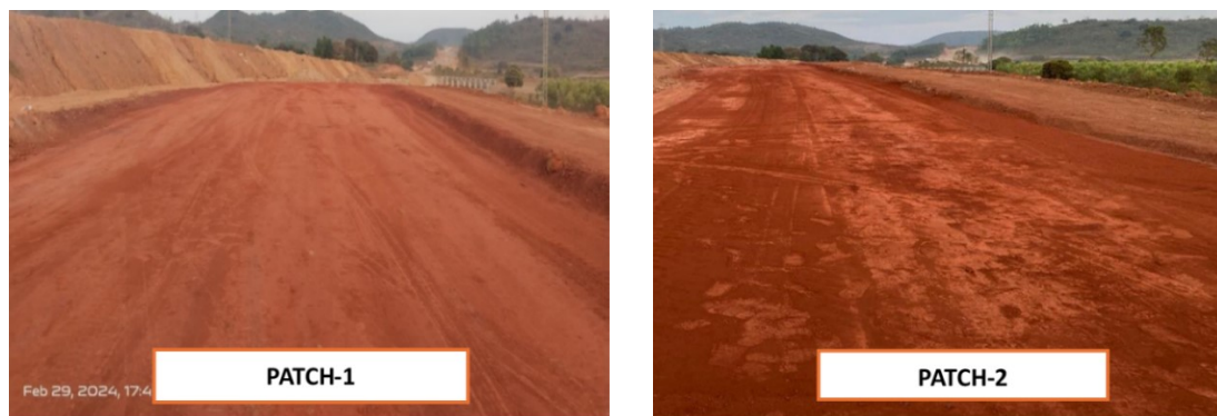
Figure 8. Red mud experimental section at chainage 289 & 290.
